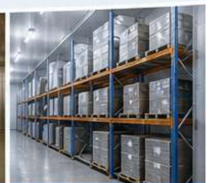
INDUSTRIAL COLD STORAGE
